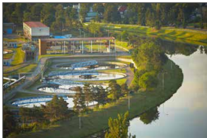
Water analysis for water treatment plants
