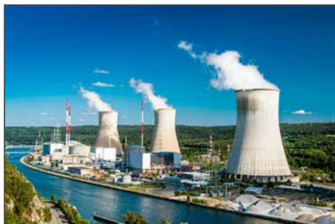
Cooling water control for power plants
