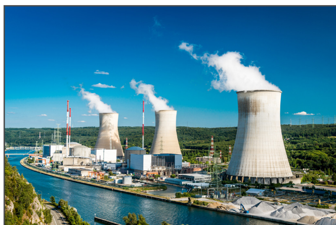
Cooling water control for power plants
