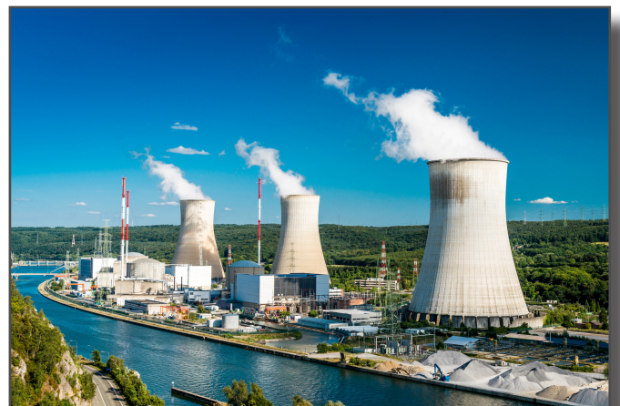
Cooling water control for power plants
