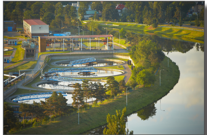
Water analysis for water treatment plants
